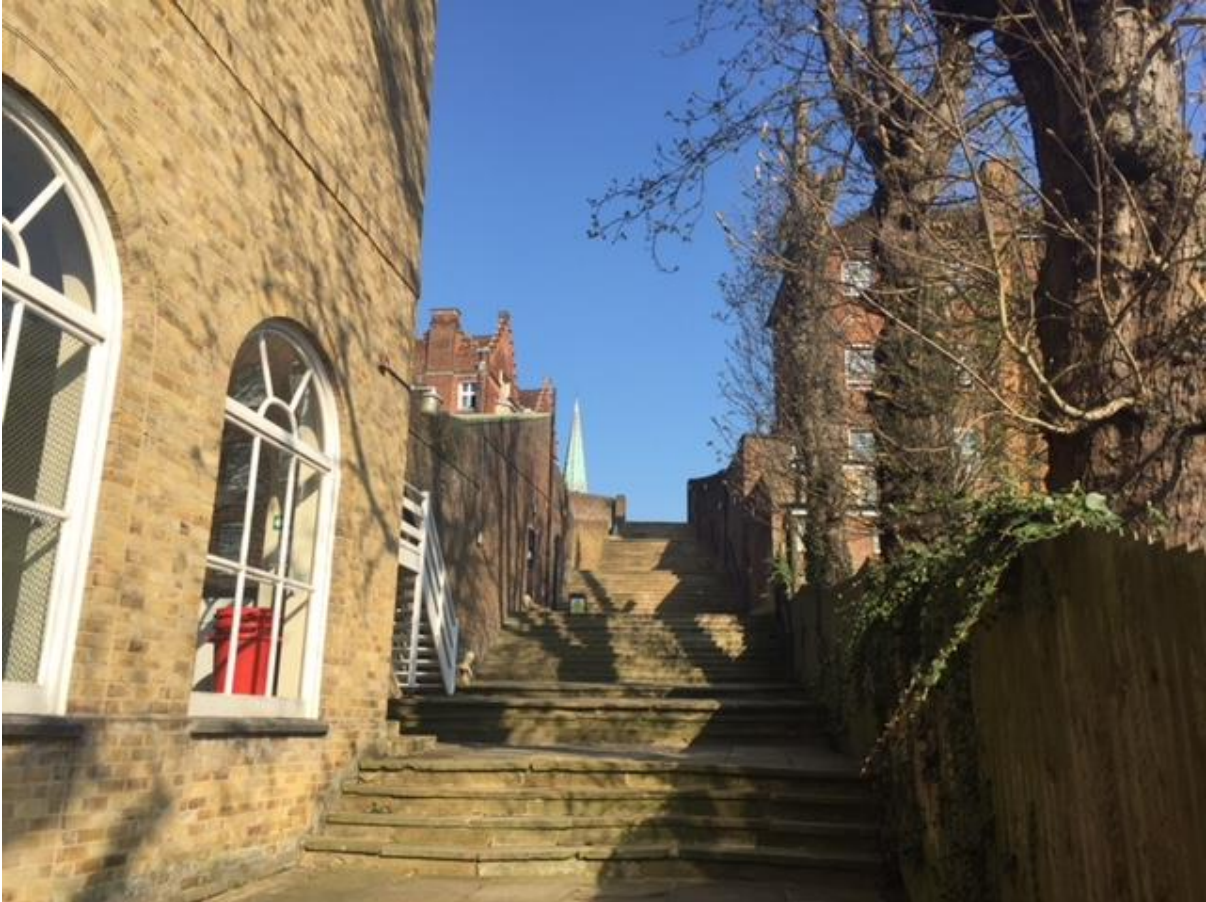
Rear elevation of host building
